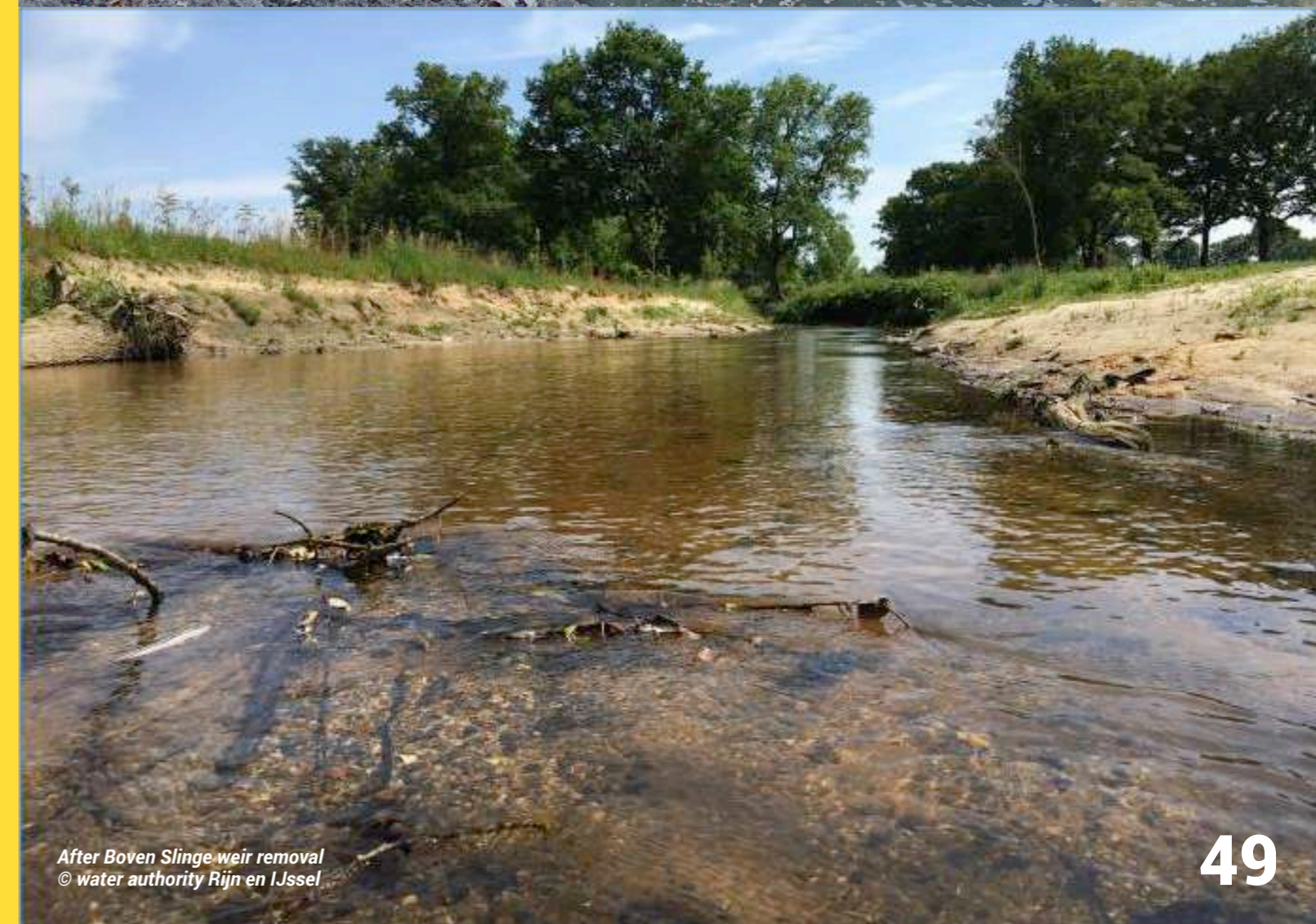
Removal works of Boven Slinge weir © water authority Rijn en IJssel
