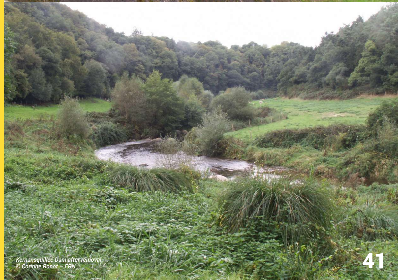
Kernansquillec Dam after removal © Corinne Ronot – ERN
